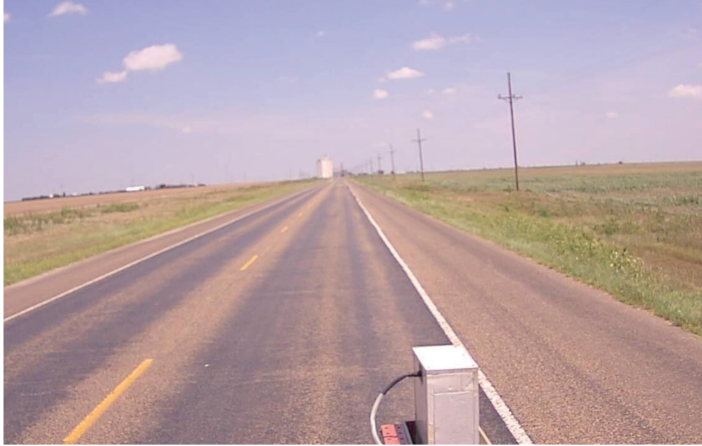
Figure 2-3. Existing Pavement Condition of SH 15 Test Sections.
