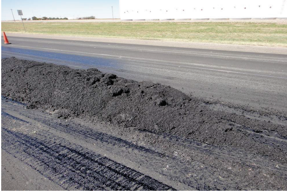
a. Big Lumps in the Asphalt Mix.
