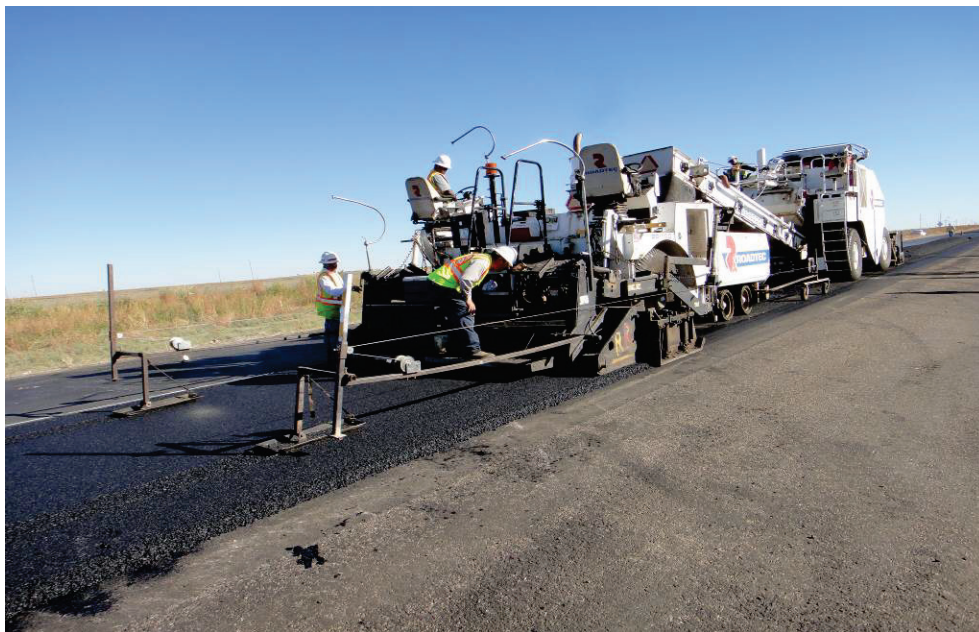
b. Paver Placing the Asphalt Mix.
