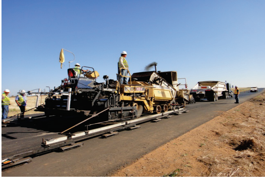
Figure 2-13. US 62 Paving Photos.
