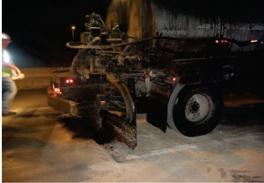
a. Tack Coat Spraying Machine.
