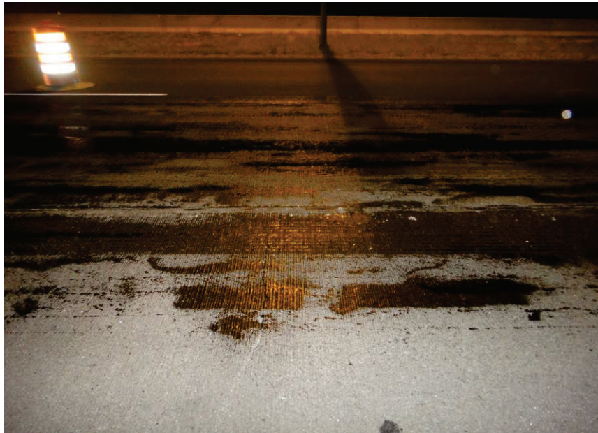
b. Pavement after Tack Coating.
