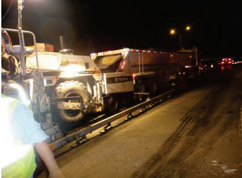
Figure 2-23. Paving Photo of Loop 820 Test Sections.
