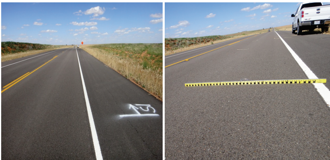
Figure 3-19. Field Survey of US 62 Test Sections.
