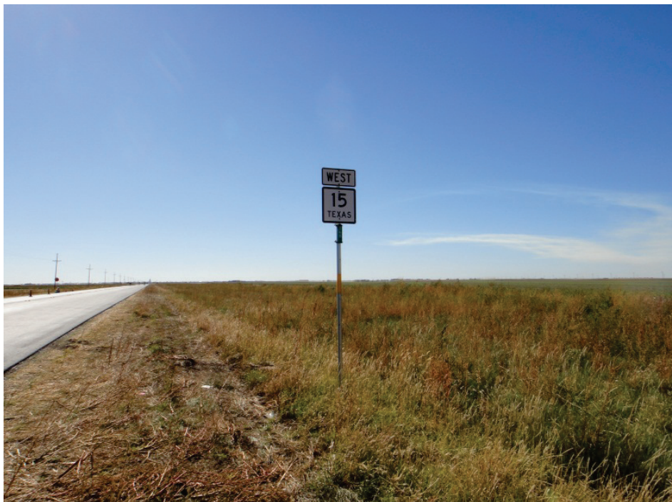
Figure 2-2. Reference Object of the Start Point for SH 15 Test Section 1.
