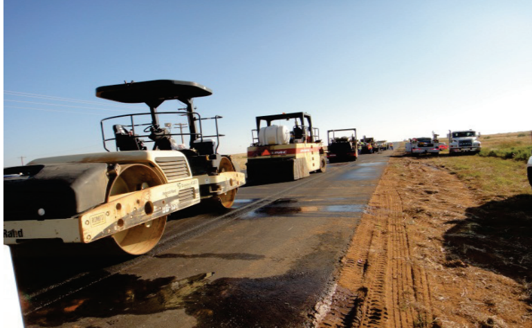
Figure 2-11. Rollers on US 62 Test Sections.
