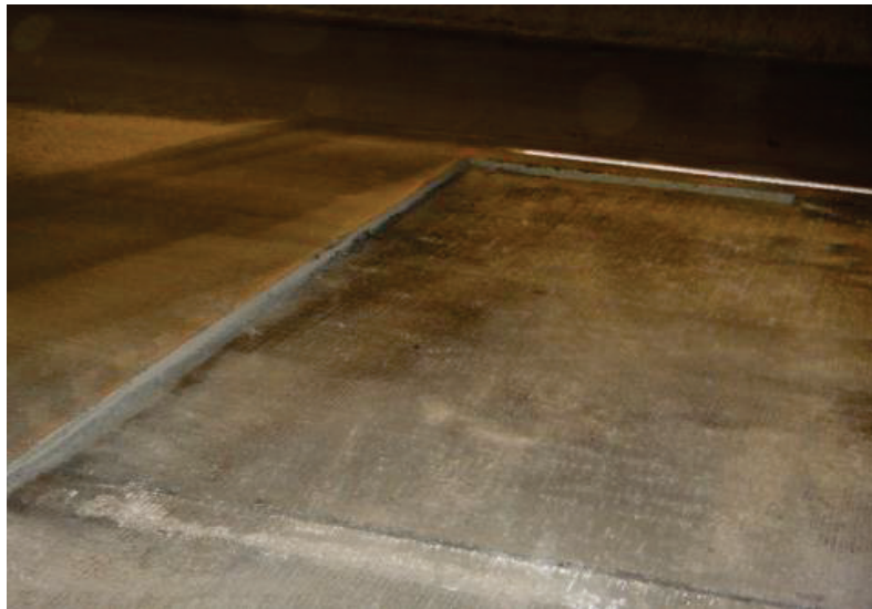
b. The Well-Prepared Edge.
