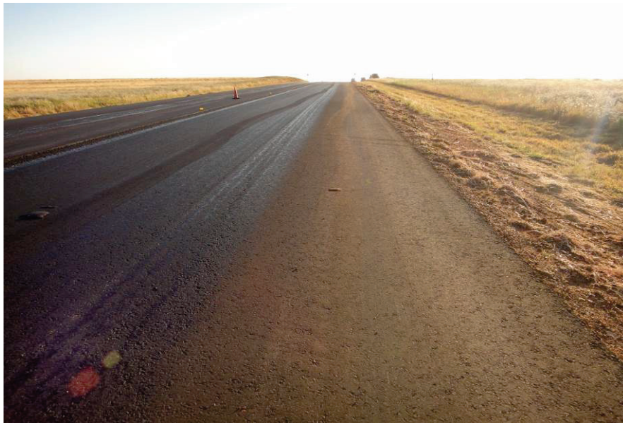
Figure 2-12. US 62 Test Sections after Tack Coating.
