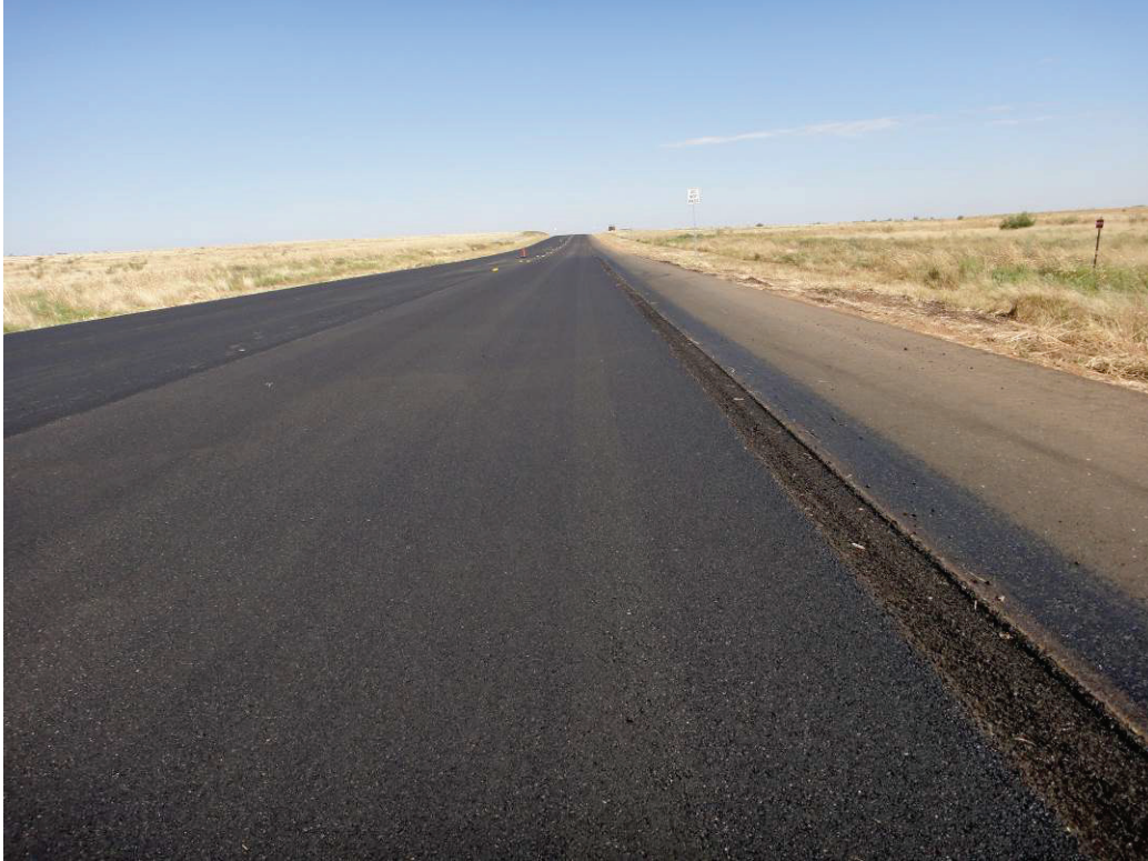
Figure 3-10. Overview of US 62 Test Sections Right after Construction.
