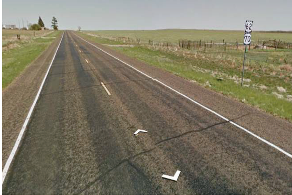
Figure 2-10. Existing Pavement Conditions of US 62 Test Sections.
