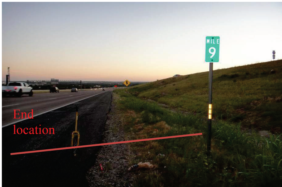
Figure 2-17. End Location of Loop 820 Test Sections.
