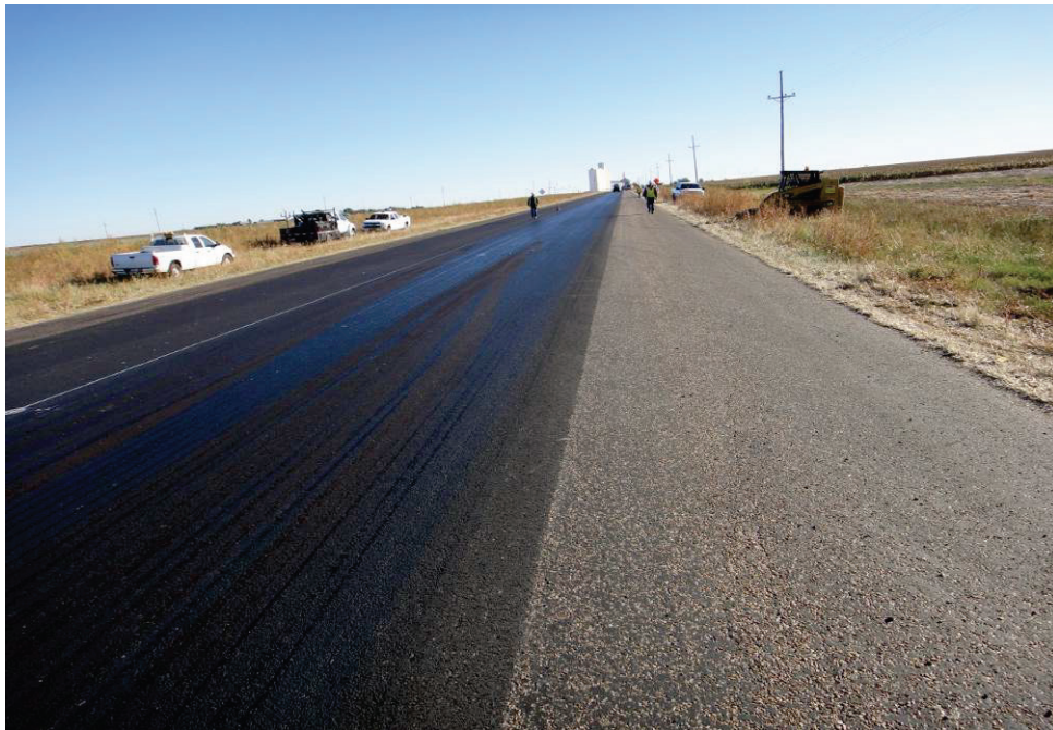
b. Test Sections after Tack Coating.
